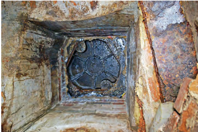
In the roof of the shelter there is an escape hatch
